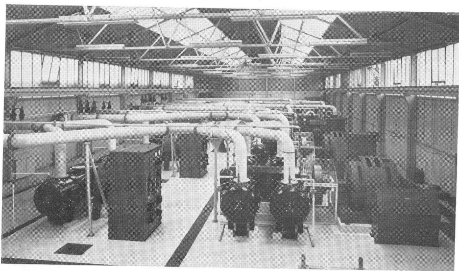
FIG. 1.1. Compressor house for construction of Clyde Tunnels, Glasgow, 1958. Low-pressure air capacity is 29,000 cu ft of free air per minute
