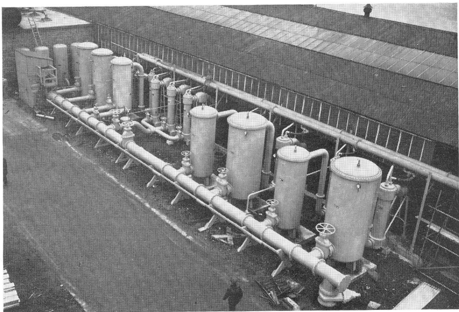
FIG. 1.3. Plant installation for cooling and purifying compressed air before delivery to working chambers
