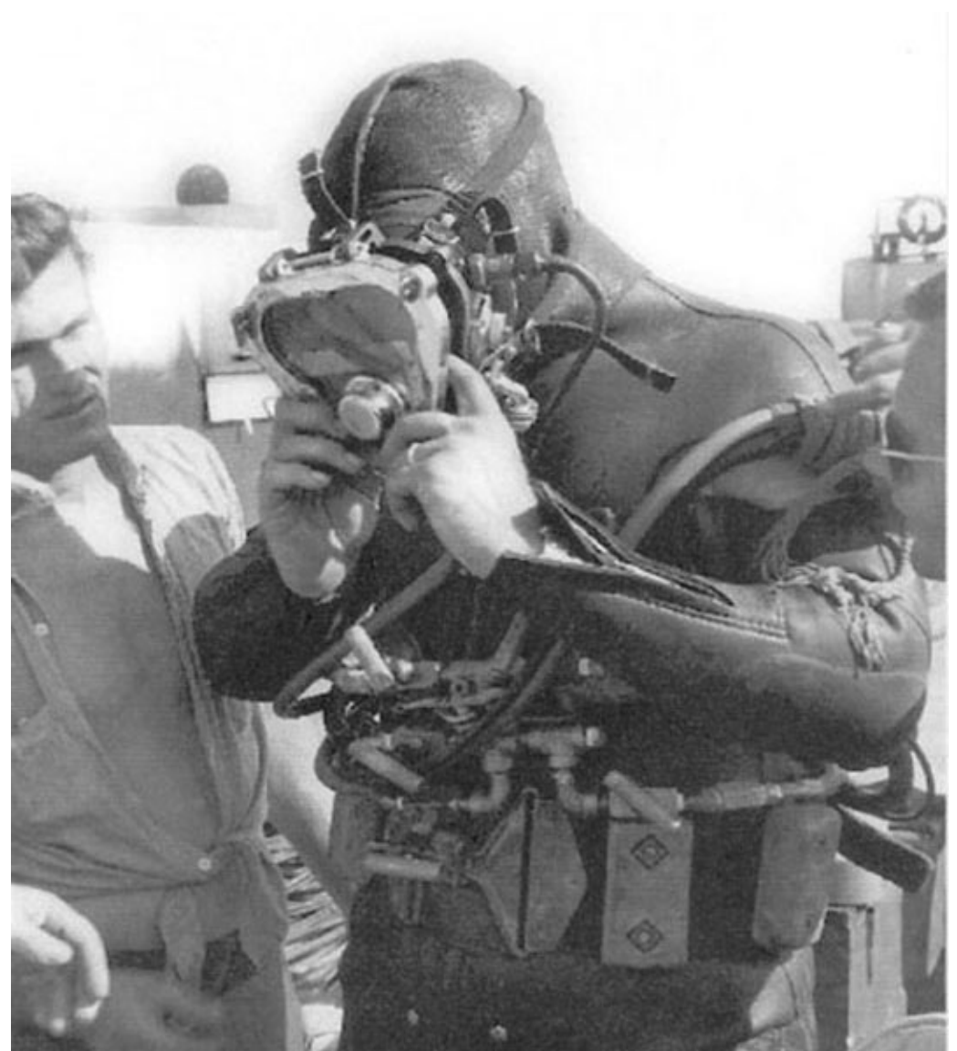
Photograph of Mike Hughes, showing the elaborate chest manifold he built to allow gas switching during the dives. The tender is 'Corky' Downer ( James Smith )
