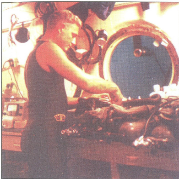
October 1965: Team III aquanaut Charles Coggeshall, Chief Gunner's Mate (DV) USN, preparing for an excursion dive, scrupulously setting up his Mark-VI diving unit. Note the TV monitoring camera outside porthole.
