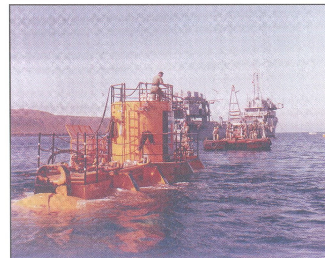
February 1969: Off San Clemente Island: Sealab III being prepared for its 610-foot descent commencing at 4:36 p.m. 15 February at a descent rate of 4 feet per minute.
