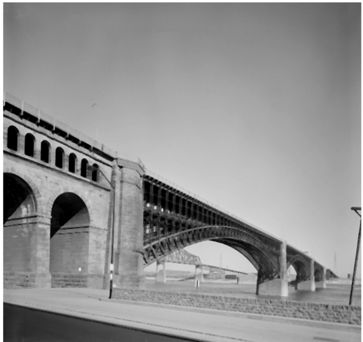
Figure 1.2 The Eads Bridge, the first bridge to span a body of water using caisson technology. (Courtesy Paul Piaget, Photographer, 1968. Historic American Buildings Survey , HABS No. MO-1190.)
