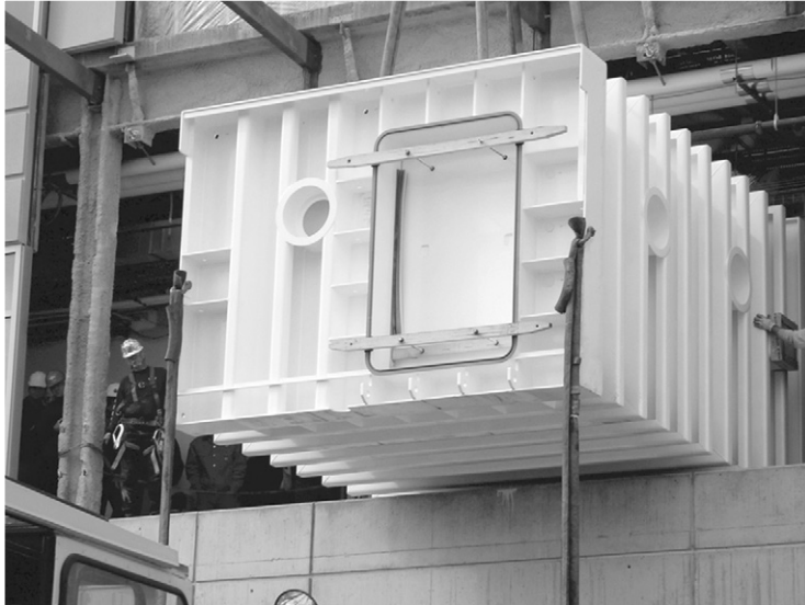
Figure 3.4 Rectangular multiplace hyperbaric chamber with external reinforcing ribs (installed 2006, Intermountain Medical Center, Murray, Utah).
