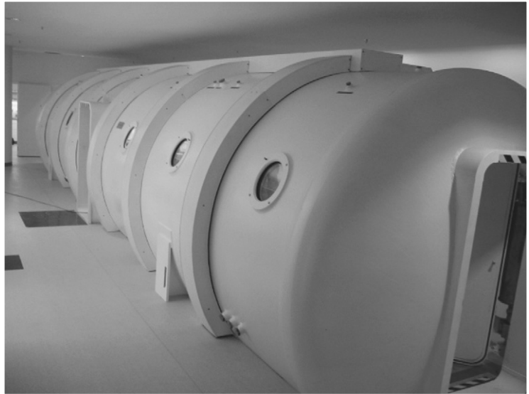
Figure 3.1 Triple-lock multiplace hyperbaric chamber with a horizontal cylinder configuration (installed 2005, Virginia Mason Medical Center, Seattle).
