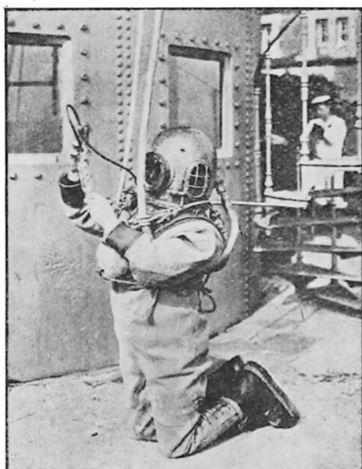
FIG. 29.—METHOD OF COLLECTING SAMPLE OF AIR IN HELMET.
