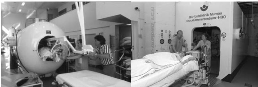
Figure 3.3-3 a. Patient transfer into a standard hyperbaric chamber with round opening b. Transportation of a critically ill patient into a hyperbaric chamber using a special transport device (Trauma Centre Murnau)
