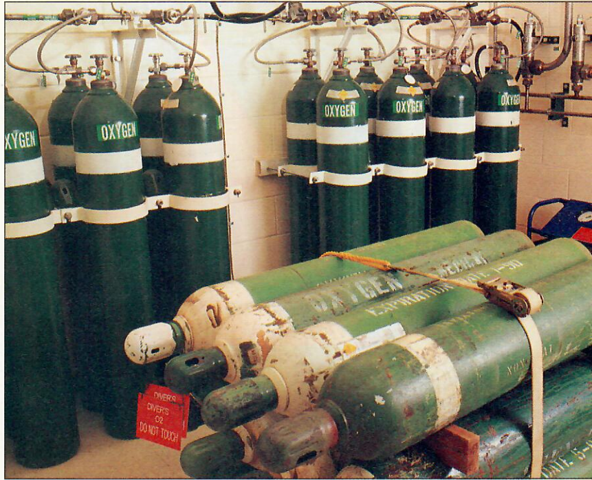
Figure 9-1. Oxygen cylinders in oxygen room at US Navy Submarine Escape Training School, Groton, CT.
