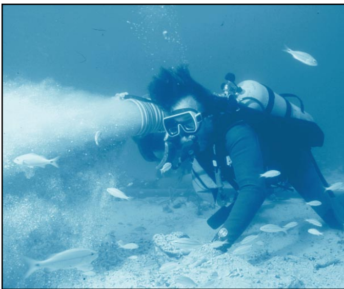
FIGURE 9.45 Backfilling with an Injection Dredge
