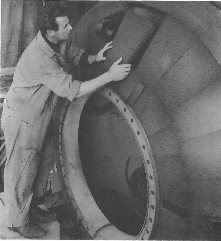
Fig. 6.34. Under-water station being insulated with glass foam.
