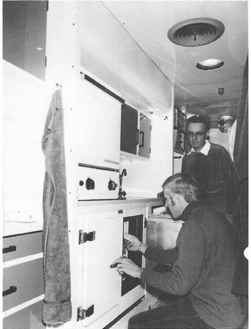
Fig. 6.47. The kitchen of the underwater laboratory Helgoland , with deep freezer, refrigerator, stove, sink, cupboard and water tank for daily consumption.
