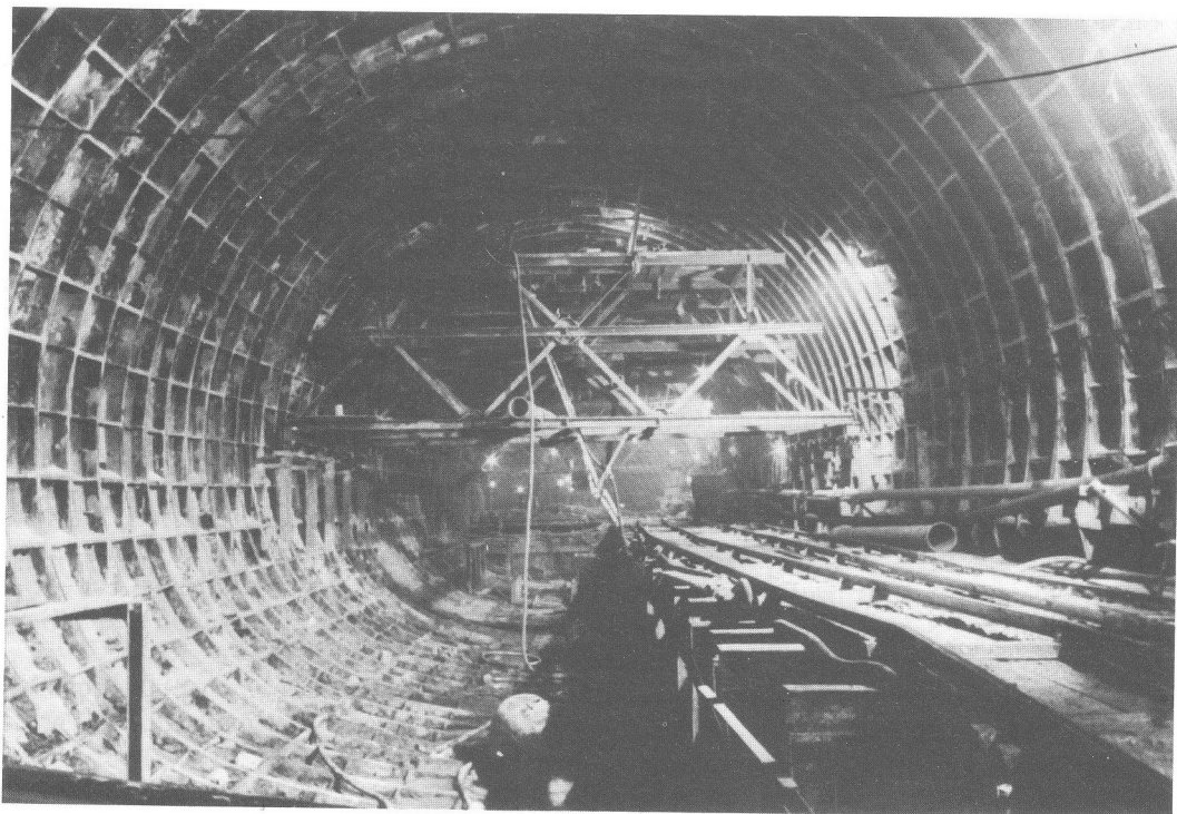
FIG. 2.2. Tunnel with elliptical cross-section. Mass Transit Railway, Hong Kong, G.K.L. joint venture
