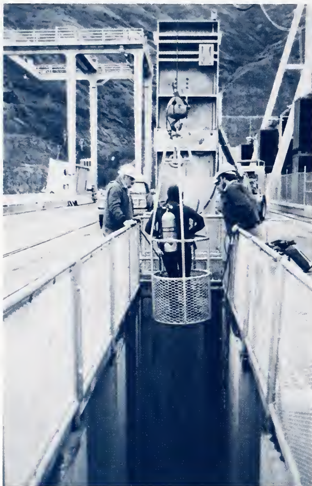
Figure 10-13 Diver Protected by Cage and Ready to be Lowered Into Dam Gatewell
