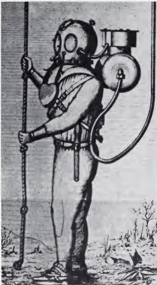
Figure 1-5 Rouquayrol-Denayrouse Semi-Self-Contained Diving Suit
