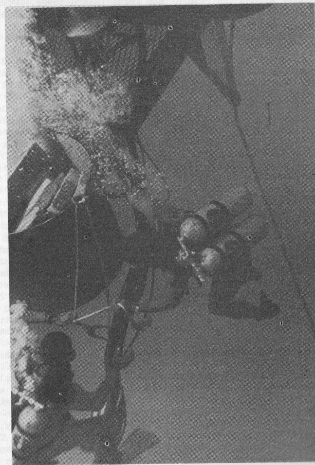
Surface support divers help rig the SEALAB I habitat.
