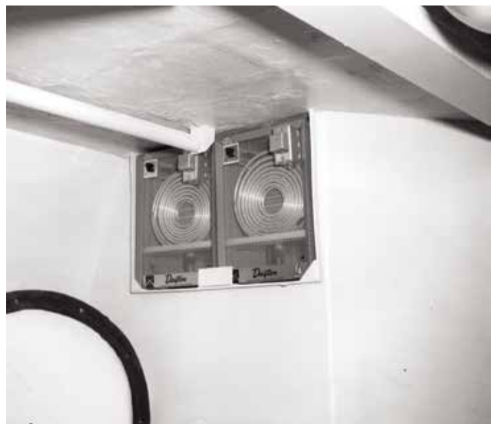
Fig. 3: SEALAB II dehumidifiers (Official photograph, U.S. Navy)
