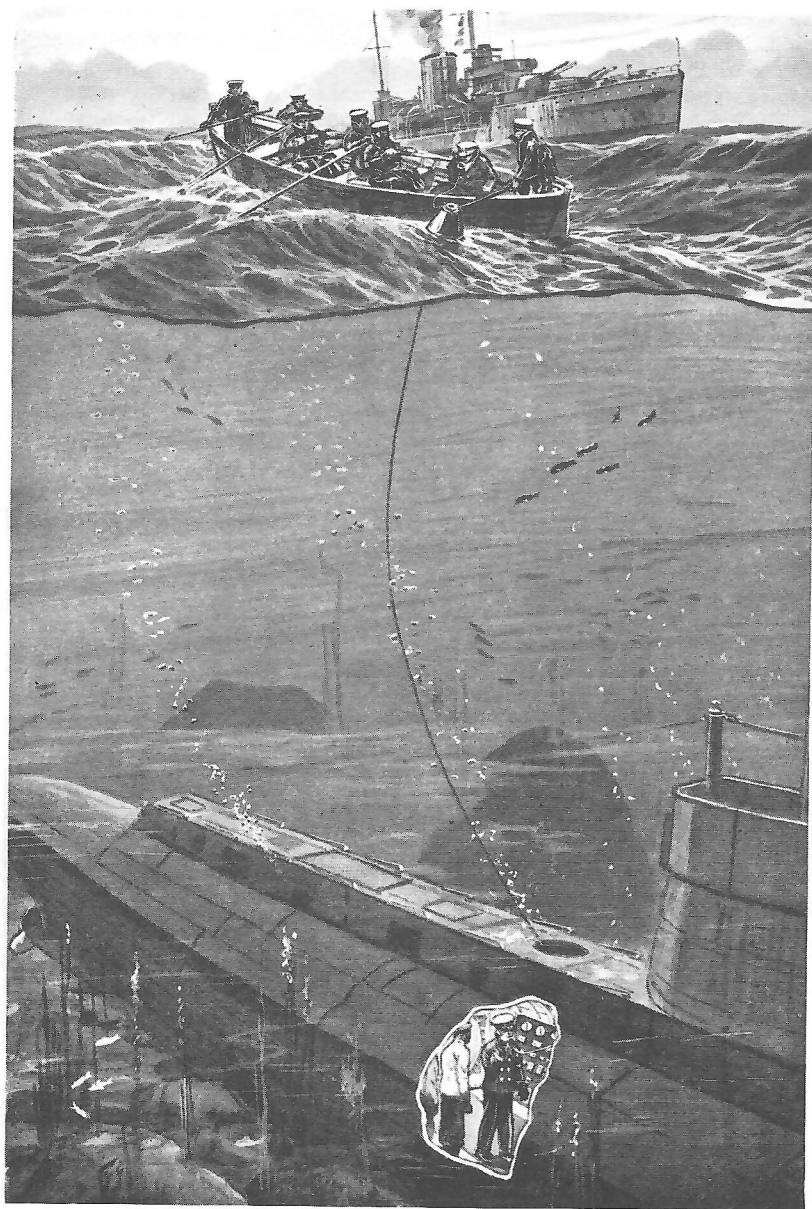
Fig. 279. Communication between submarine and surface by means of telephone-buoy
