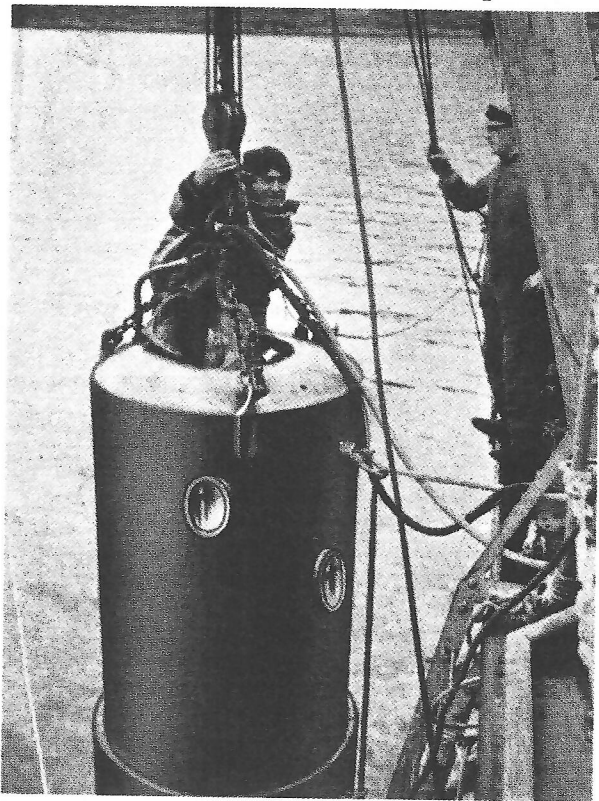
Fig. 128. R. H. Davis's submersible decompression chamber; diver emerging after decompressing
