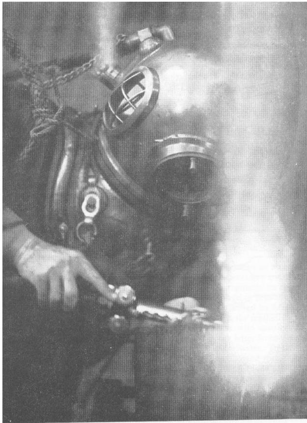
Fig. 185. Underwater cutting in operation
