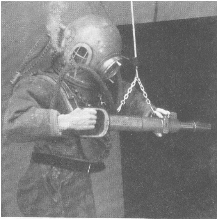
Fig. 193. Diver using Cox gun under water
