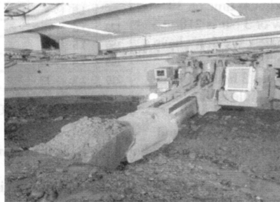
Figure 11. Robot excavator inside the caisson.
