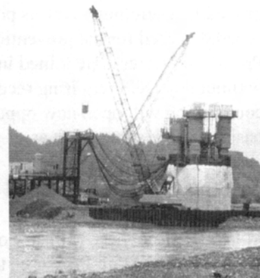
Figure 7. Caisson work at Ohigawa River, 1977.
