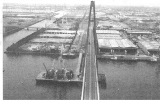
Figure 4. Caisson for the new bridge as seen from the old Meiko West Bridge.
