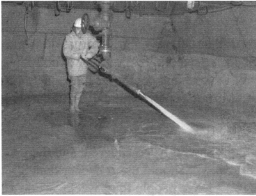
Figure 13. Water cannon for ground removal inside a caisson.
