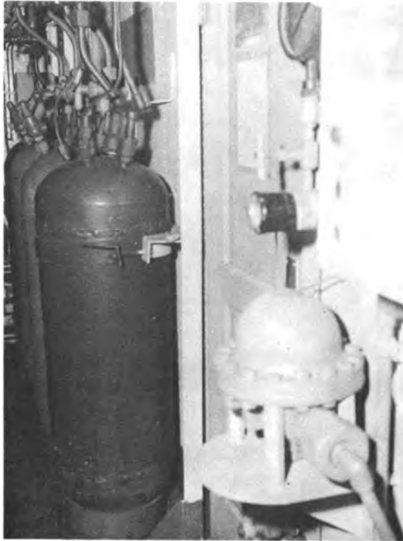
FIGURE 2-38.—He-O 2 and O 2 volume tanks.
